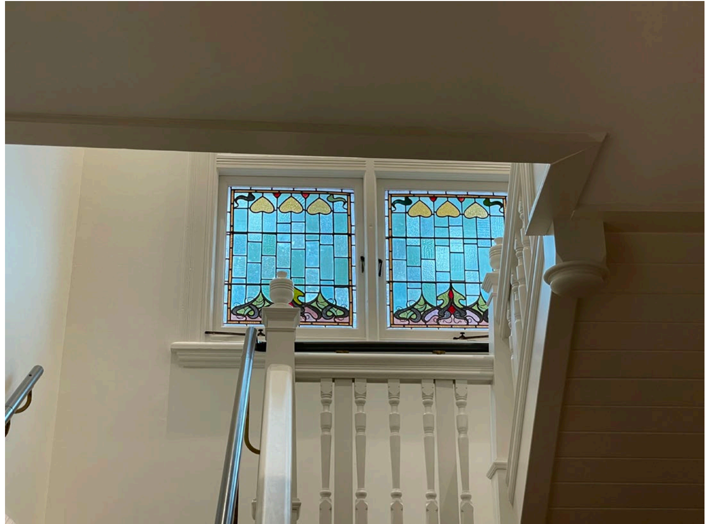
View from ground floor to stair landing, showing balustrades and timber handrails. (Source: GML Heritage)
